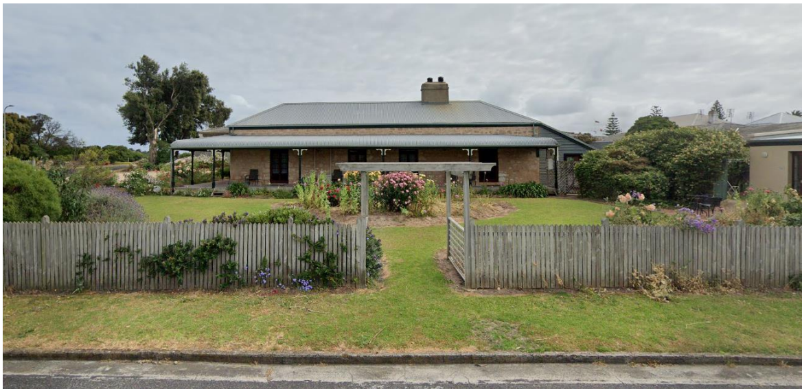
Southern elevation showing French doors and lean-to, 2020.
