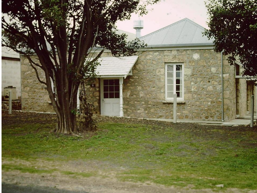
Front façade of Former Government Residency facing west, c.1982.
