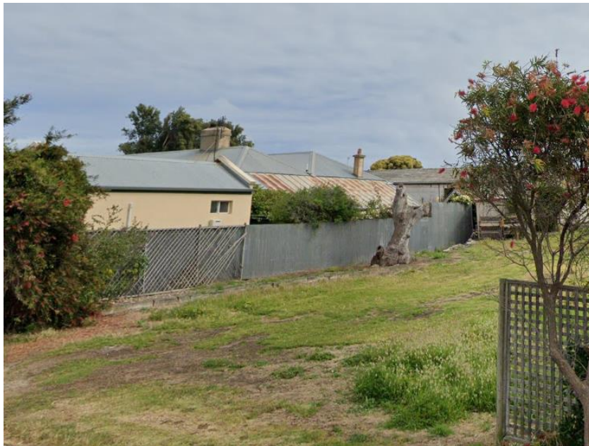
The roof of the lean-to, 2020.
