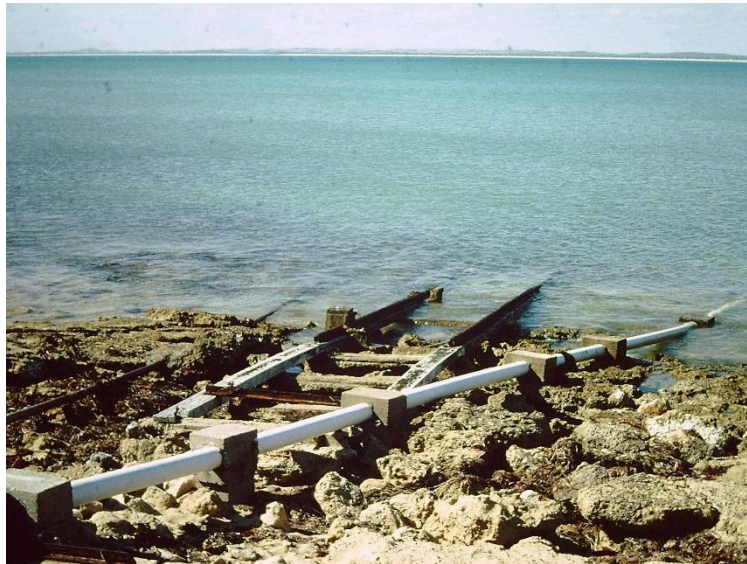
The remains of the original slipway, c.1983
