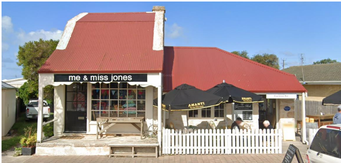
Front of Attic House showing shop and attached dwelling, September 2023.
