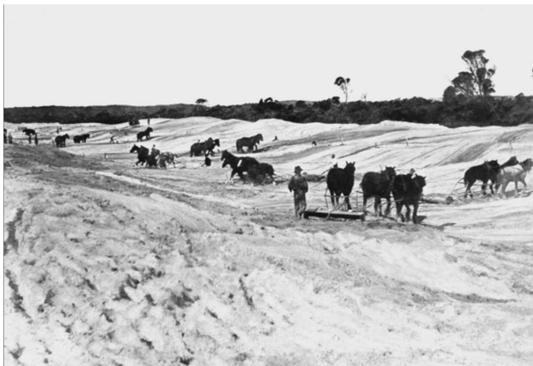
Horses being used to assist dig Drain L, which is located near Robe, c.1917.
