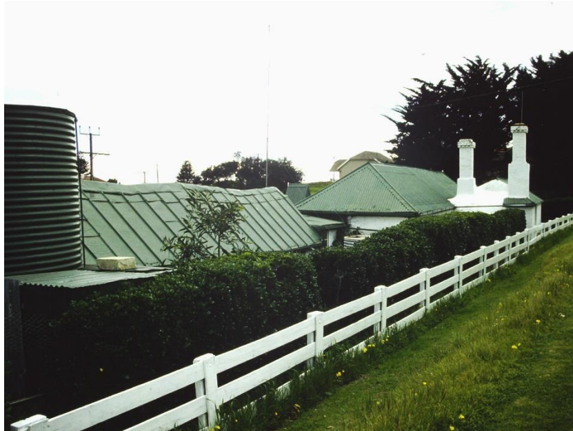
Roof of the 1840s cottage (left), c.1982.
