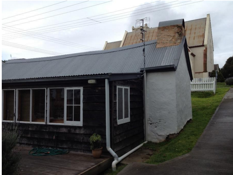
Rear of the 1840s cottage showing the eastern elevation, c.2012.
