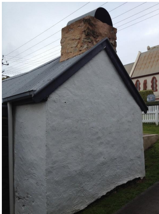
Eastern elevation of the 1840s cottage showing chimney, c.2012.
