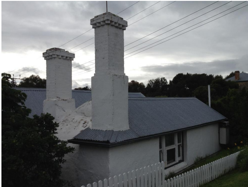
Two chimneys built of brick and stone on the c.1853 addition, c.2012.
