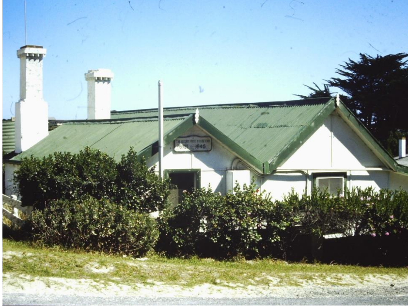
Front elevation of the c.1853 section of Granny Banks' Cottage, c.1982.
