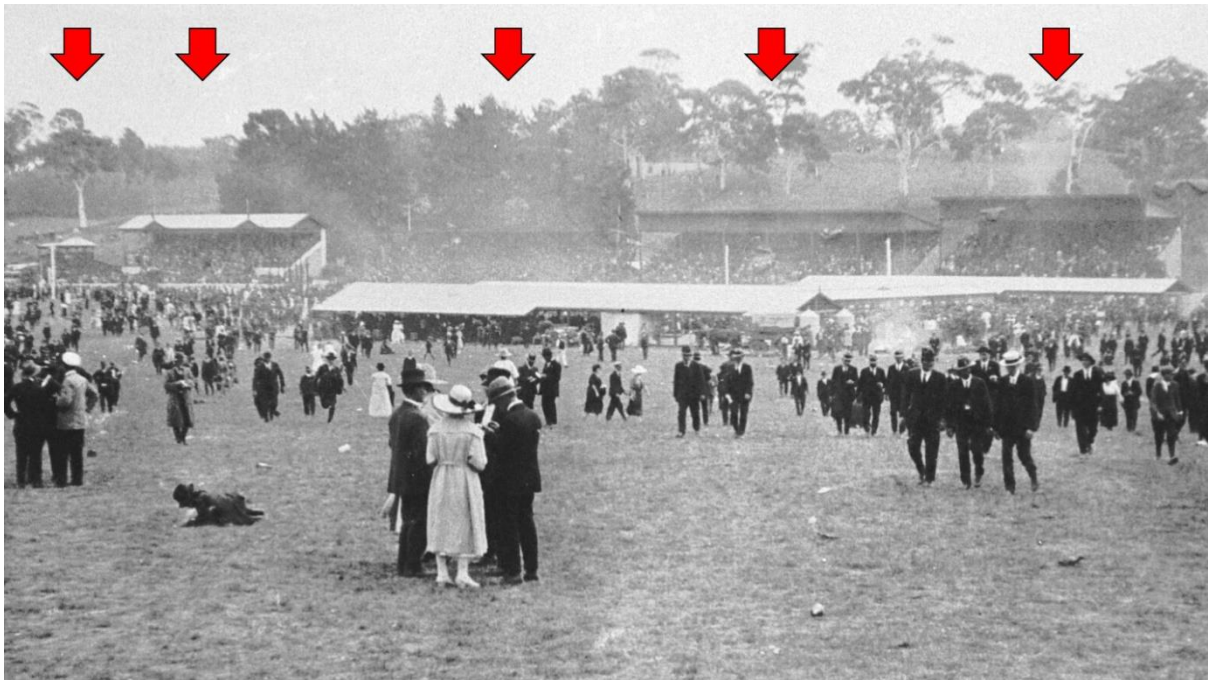
Oakbank Racecourse c.1922, showing (background buildings left to right) second Steward's Stand (1910, demolished or considerably altered), second Members' Stand (1898, extant, now known as the Shillabeer Stand), Grandstand (1885, extended 1891, demolished c.1923), Stand (1914, extant, now known as the John Glatz Stand), second Derby Stand (1911, extant), note gable-roofed totalizator buildings in front of the stands on the flat.
