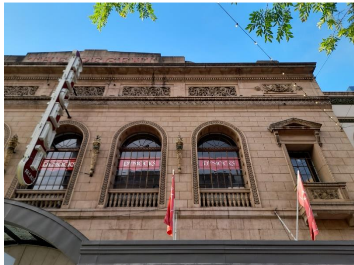
Former Regent Theatre (facade) detail, 6 October 2023
