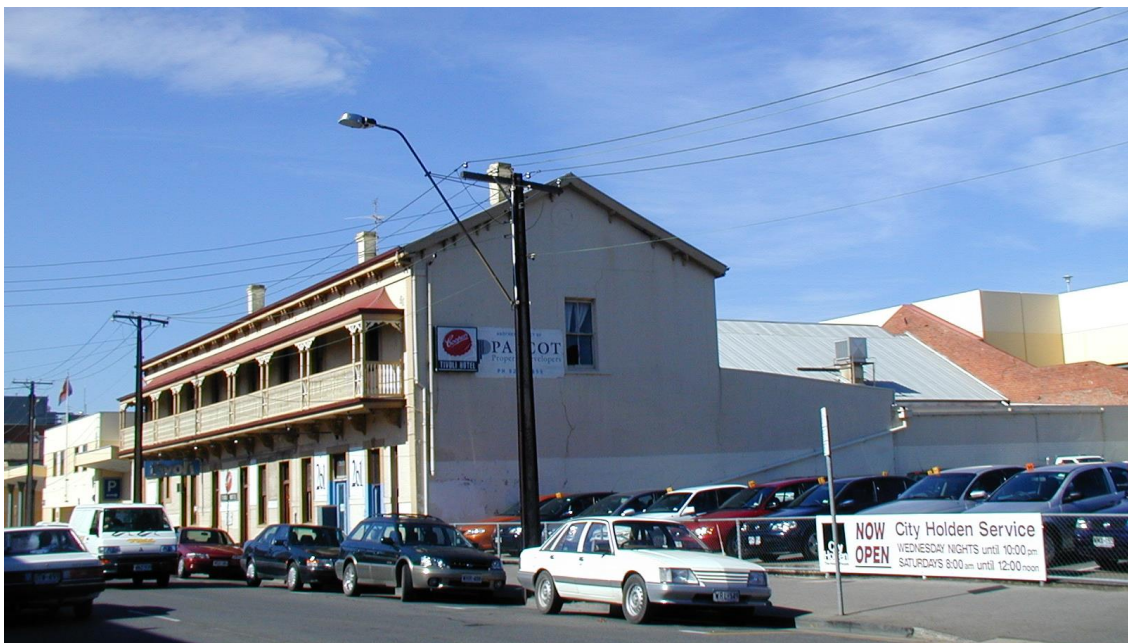
Tivoli Hotel, with roof and rear wall of theatre/ballroom behind
