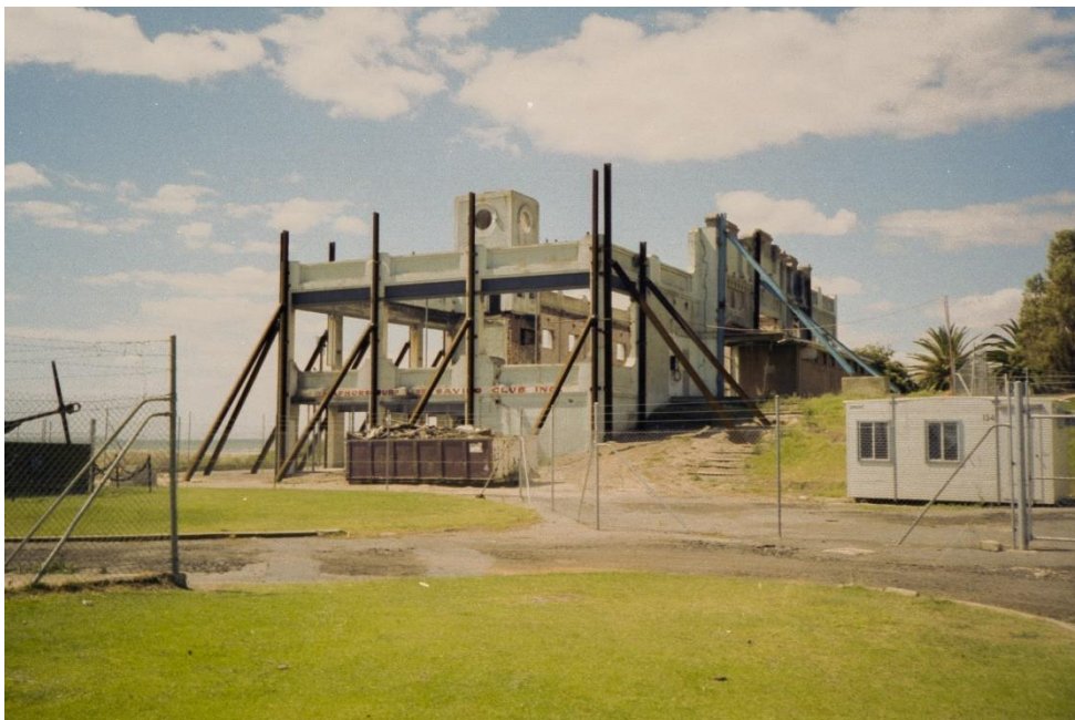
The four original walls and tower salvaged following the fire, 1994.
