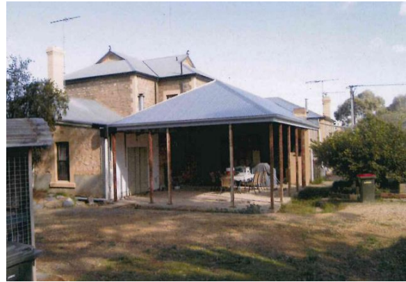
The rear extension during construction in June 2010.
