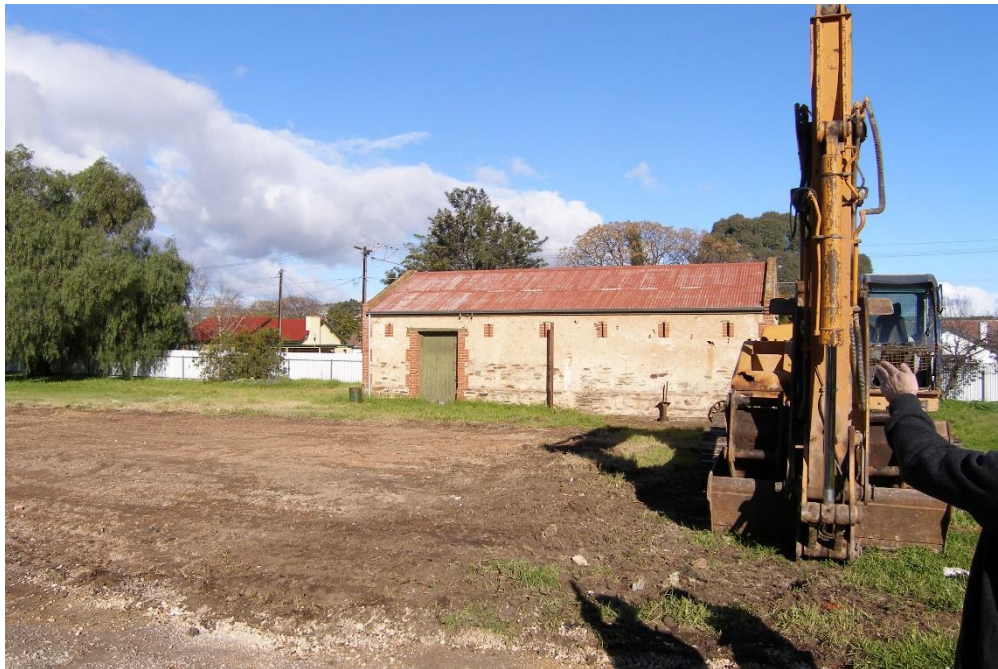
Northern elevation of Outbuilding Two, 26 June 2007.
