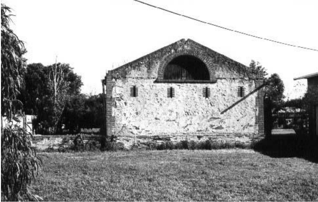
Eastern elevation of Outbuilding Two, July 1993.
