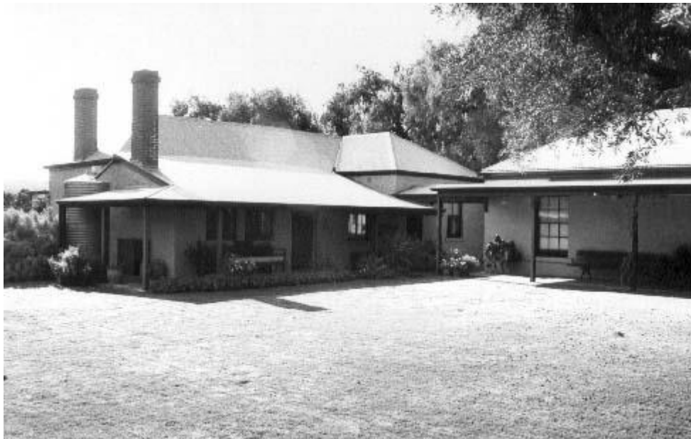
Southern elevation of the cottage showing lean-to extension and verandah. According to the owner, the building to the right was erected in the 1980s.
