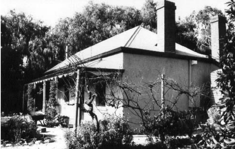
Western elevation of the cottage, July 1993.
