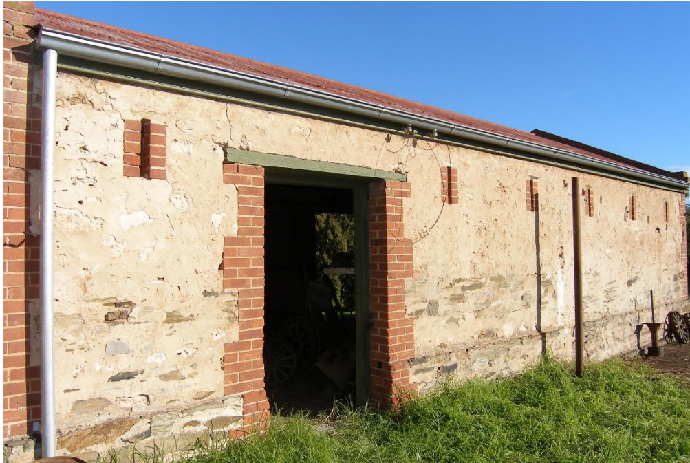
Southern elevation of Outbuilding Two, 26 June 2007.
