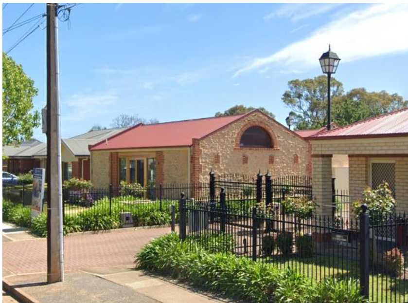
Eastern elevation of Outbuilding Two, October 2021
