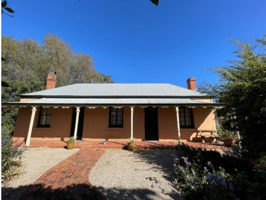
Northern elevation of the cottage, September 2023.
