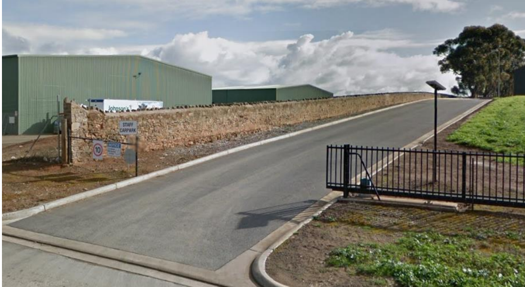
Bluestone Wall along south-east boundary.
