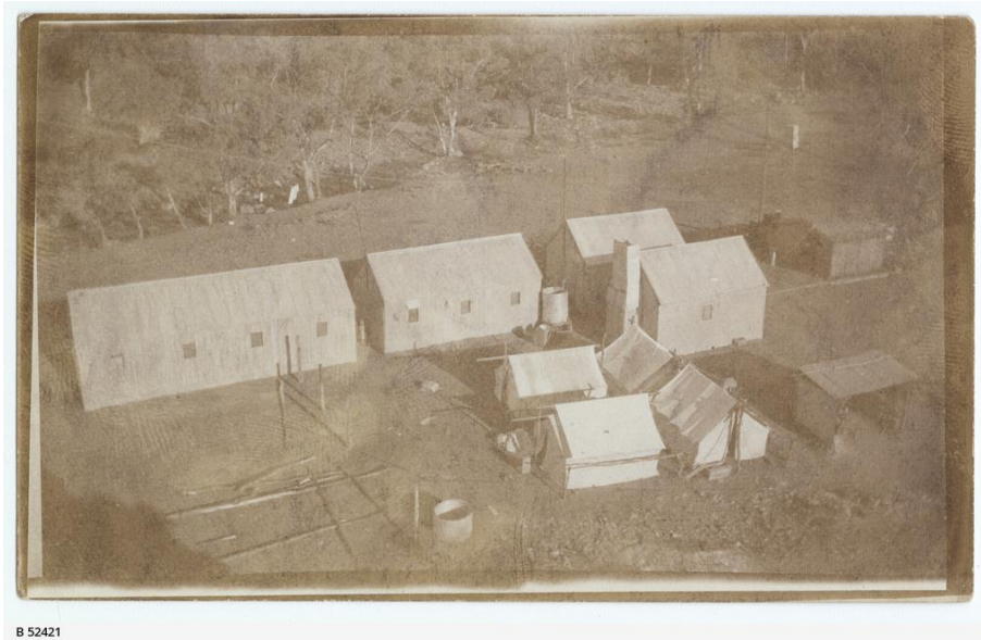
'The Camp accommodation at Paralana Springs.'
