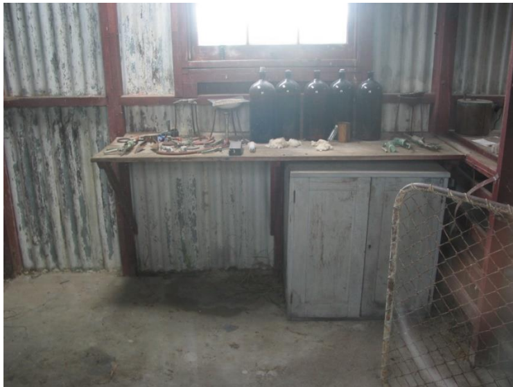
Inside of the shed facing towards the east, April 2003.
