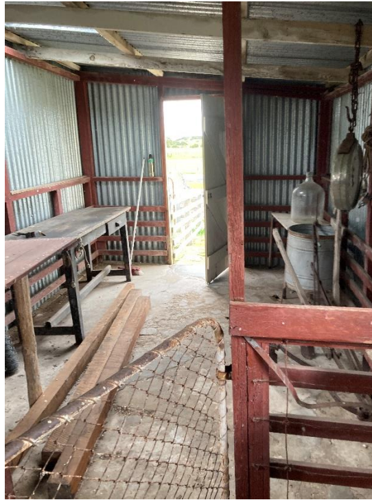
Inside of the shed facing the front entrance, 2022.
