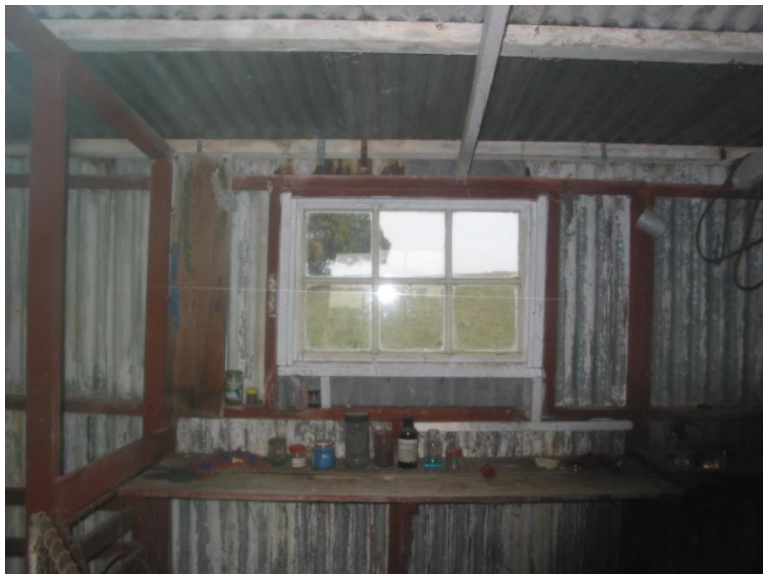
Inside of the shed facing towards the west, April 2003.
