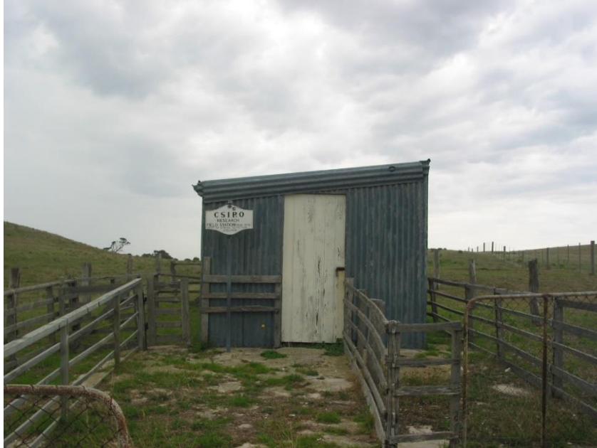
Entrance to the shed showing entrance, signage, a section of the concrete yard, timber fencing, and steel-framed wire gates, April 2003.
