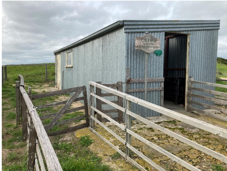
Front and western side of the Research Station showing both doorways, wooden fencing and concrete surfacing, 2022.
