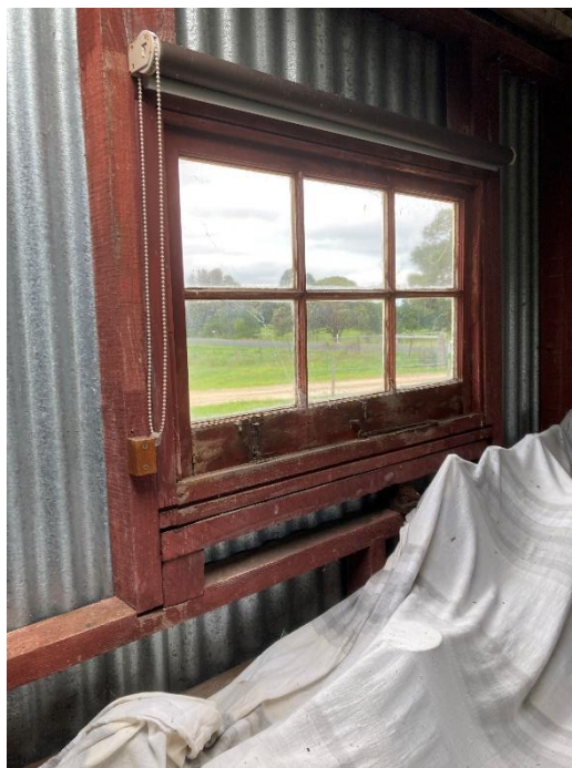
Detail view of the window on the eastern side, 2022.
