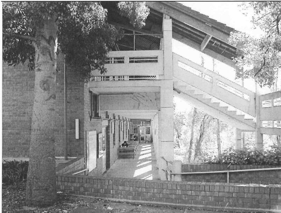
Stairs, east elevation
