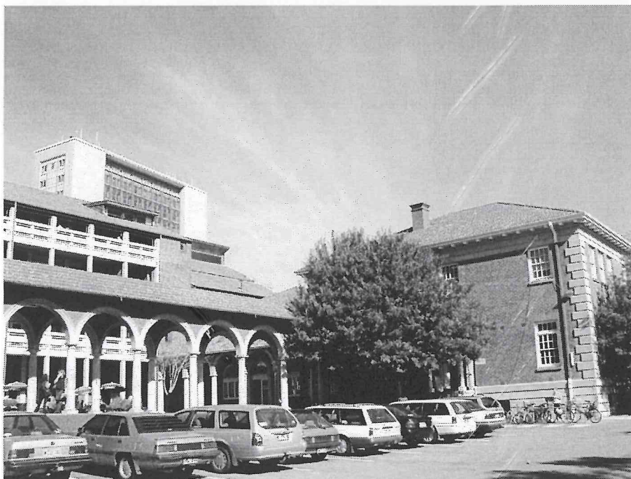
Cloisters & Lady Symon Building
