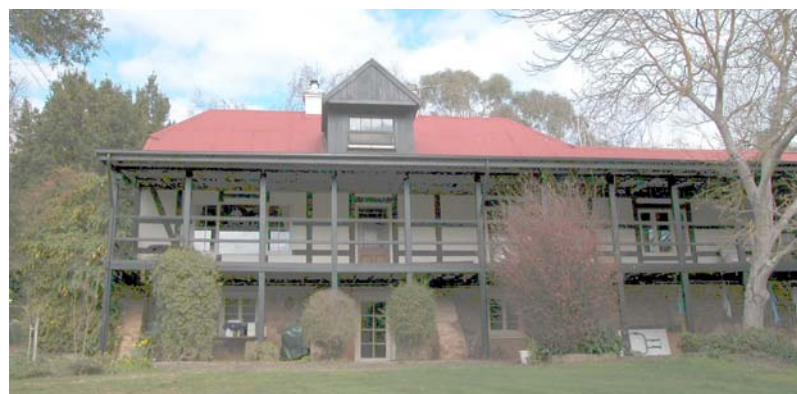
Oakside Park Stud, front elevation of house showing later alterations
