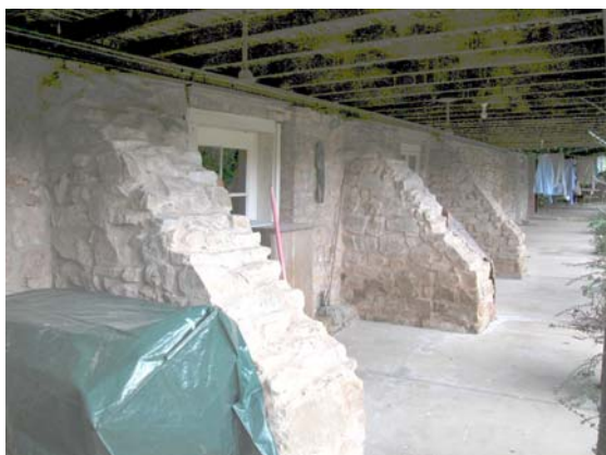
Oakside Park Stud, basement detail of fr Paech house, 2004 – note substantial stone buttresses
