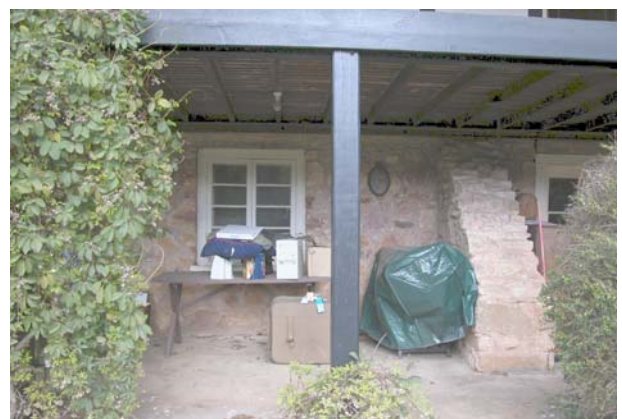
Oakside Park Stud, basement detail of fr Paech house, 2004 – note substantial stone buttresses
