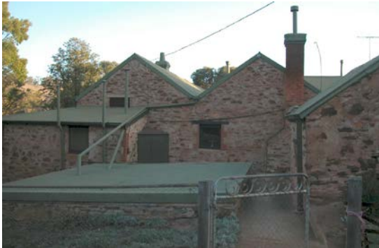
Rear of house, tank & outbuilding (possibly dairy?) looking S.
