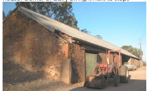
Winery building 1 – looking SE Known as the cellars
