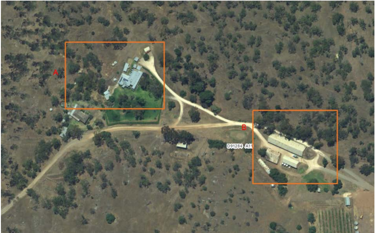
Site Plan of House and Winery Complex, indicating relationship of significant components
