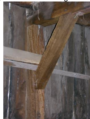
Detail of Slab Barn No 1 interior
