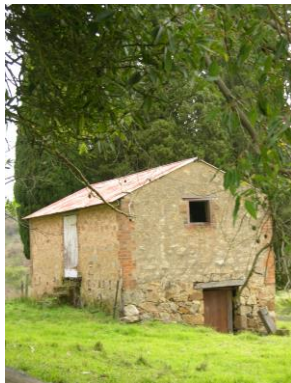
Stone outbuilding looking north from track
