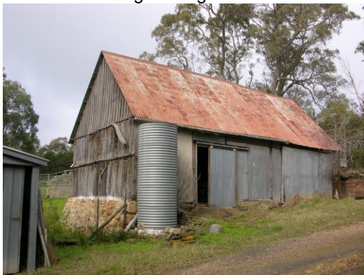
Slab Barn No 1 (looking south)
