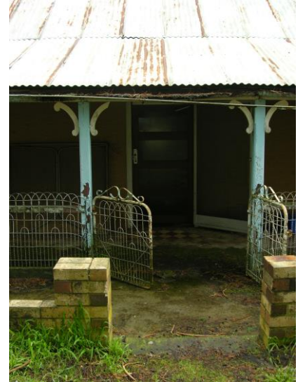
Front door of 1840s house (SW façade)
