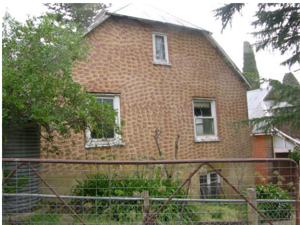
Eastern façade looking west from track
