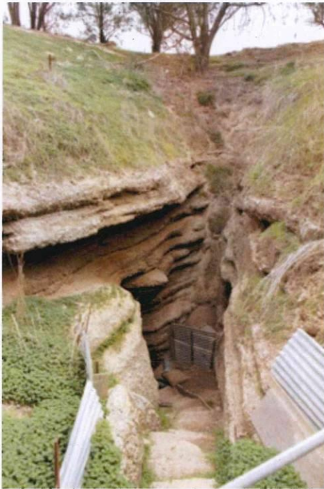
Corra Lynn Cave entrance: note erosion and stabilising work undertaken by cavers and landowner
