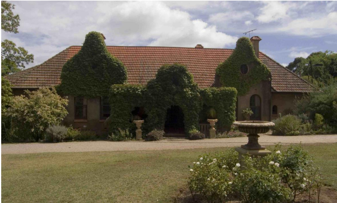
Scammell residence, Beaumont, looking north
