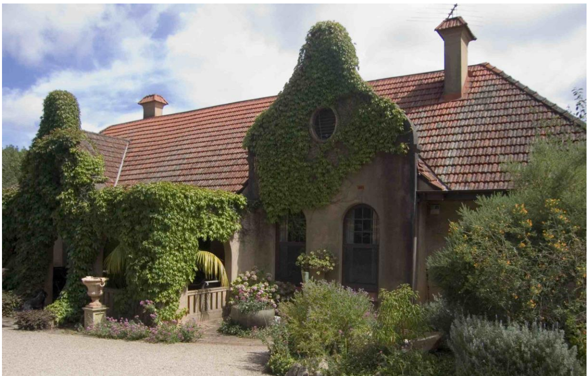
Scammell residence, Beaumont, looking north-west
