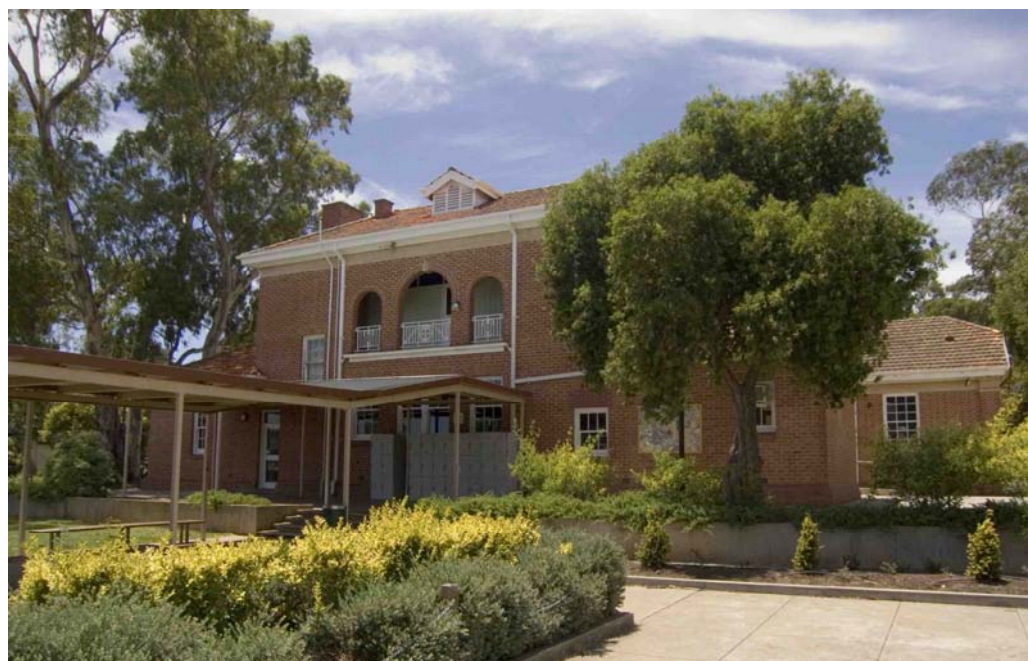
Original School Building/Headmaster's Residence, Urrbrae Agricultural High School
