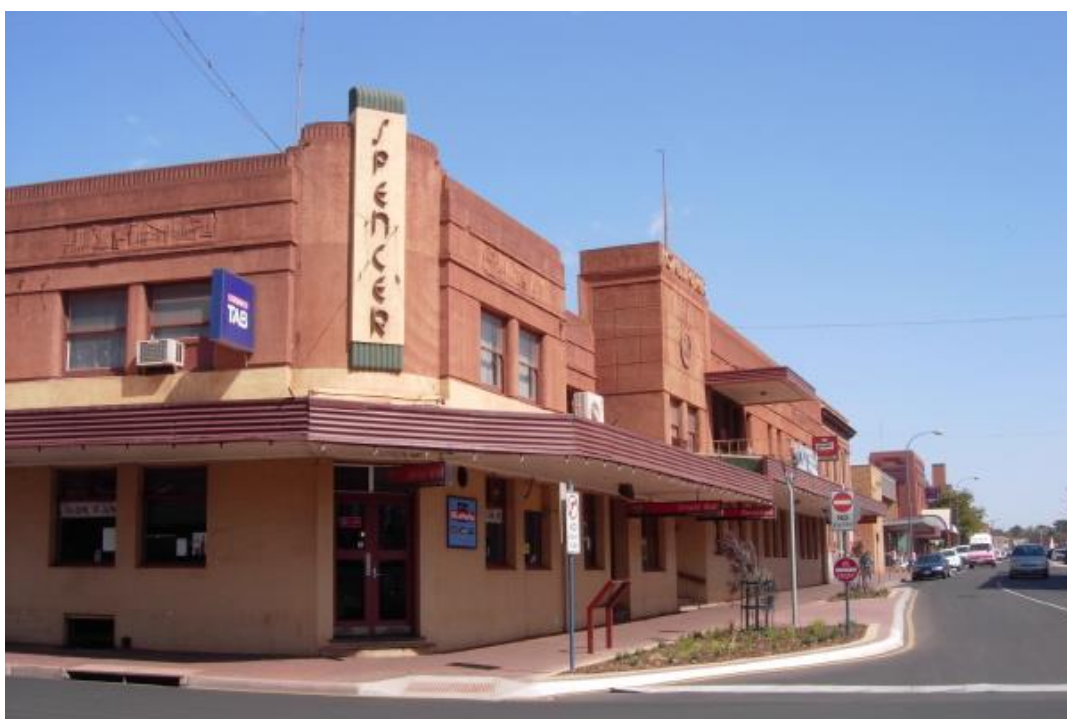
Spencer Hotel, looking down Forsyth Street to Bay View Hotel
