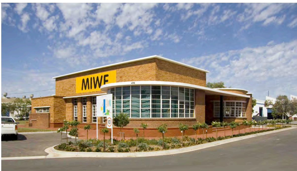
Former Tubemakers Administration Building 2, looking south-west
