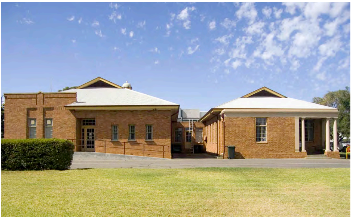
Former Tubemakers Administration Building 1, looking south
