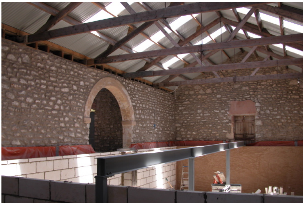
Wool Store, interior undergoing renovation
