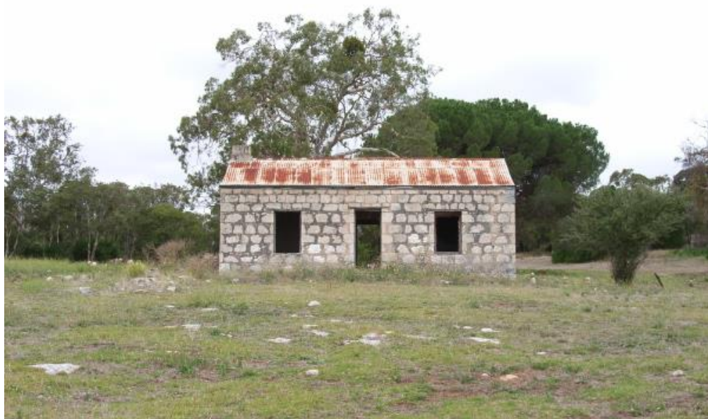
Blackford Reserve, cottage east of Rowney Road
