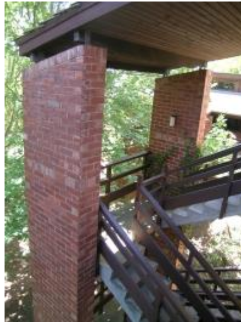
Amenities Wing stair, looking NW from balcony (image: Hurst 2009)
