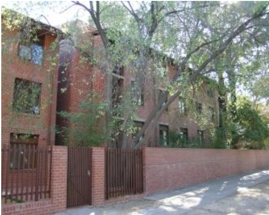
Mackinnon Parade streetscape; looking north east to 1968 Residential Wing . (Note the 2008 Residential Wing addition shown on extreme left.) (image: Hurst 2009)
