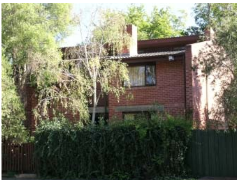
Master's House, Mackinnon Parade elevation, looking north (image: Hurst 2009)
