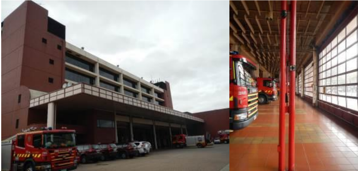
Adelaide Fire Station, 81-129 Wakefield Street Adelaide, View from South West & Interior (Simon Carter, July 2014)
