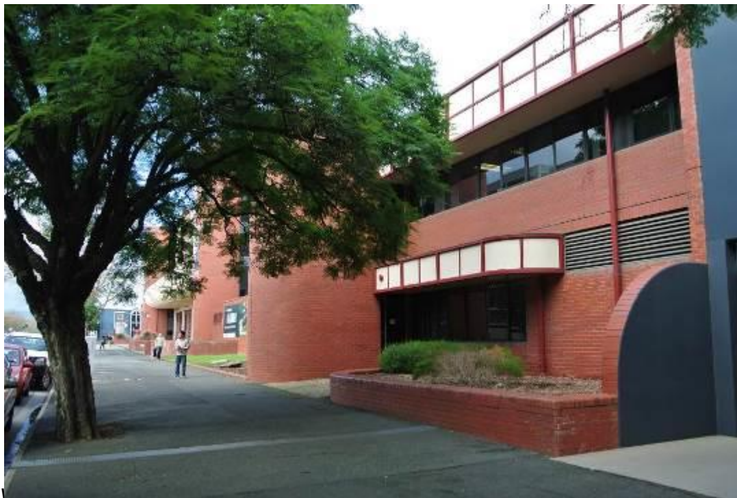
Adelaide Fire Station, 81-129 Wakefield Street Adelaide, View of western office building from north-west (Hamish Angas, July 2014)
