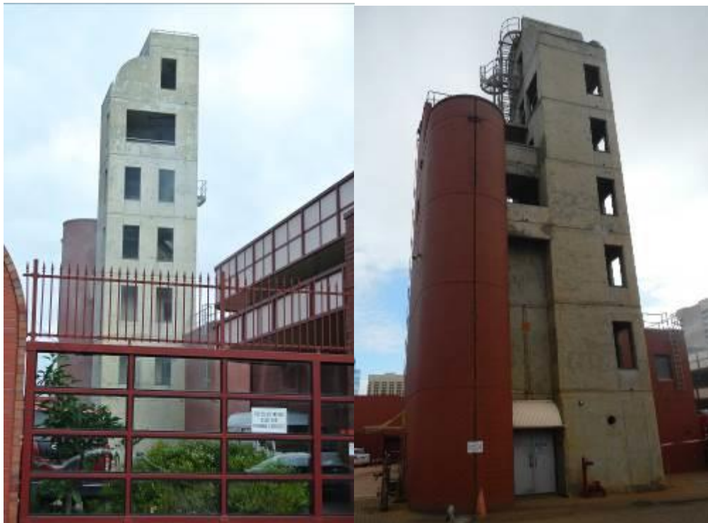
Adelaide Fire Station, 81-129 Wakefield Street, View of training tower from north & east (Hamish Angus, July 2014)
