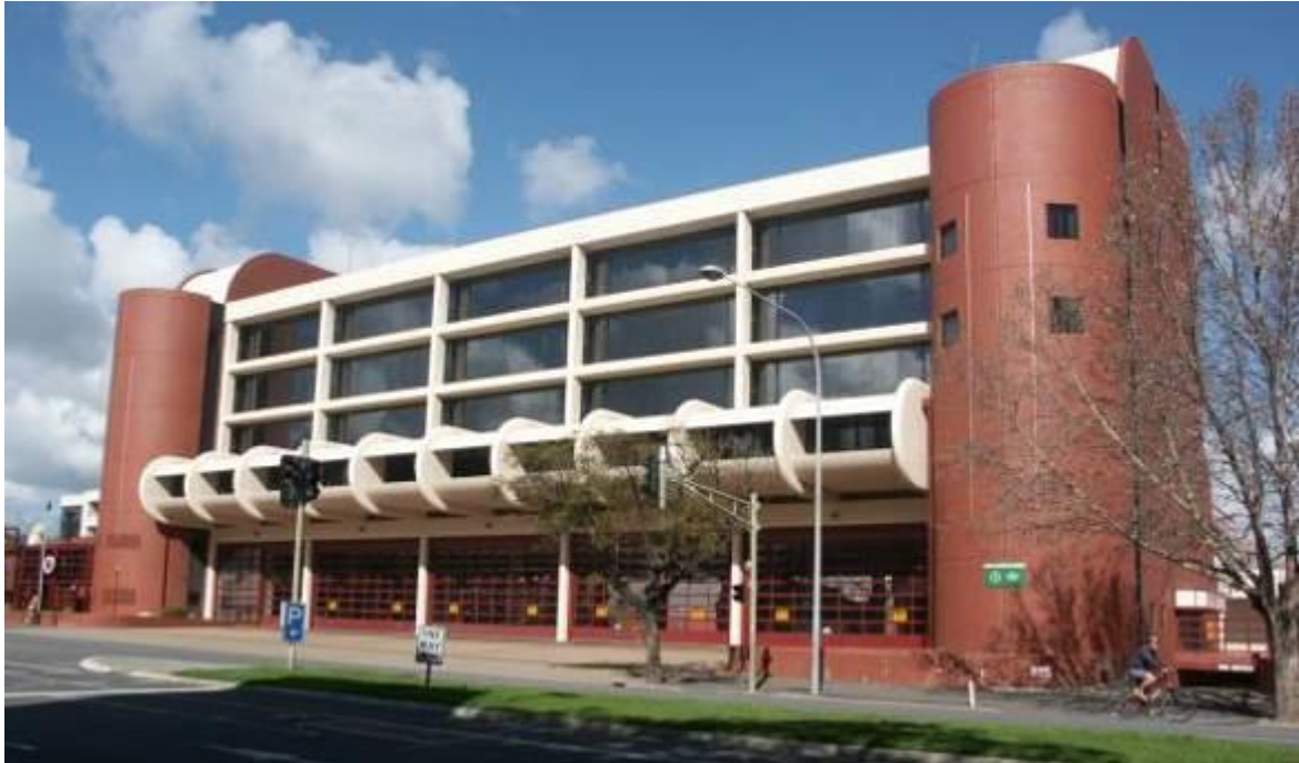
Adelaide Fire Station, 81-129 Wakefield Street Adelaide, View from north (Hamish Angas, July 2014)
