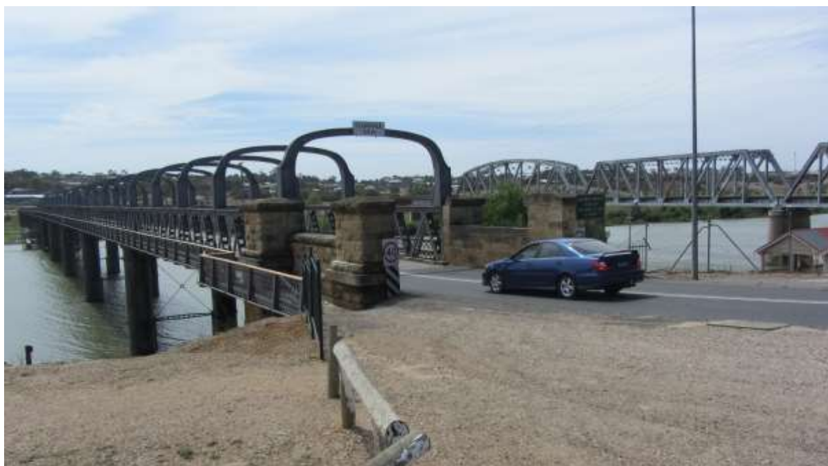
The Murray Bridge (SHP: 10287) Murray Bridge Transport Precinct, Murray Bridge
