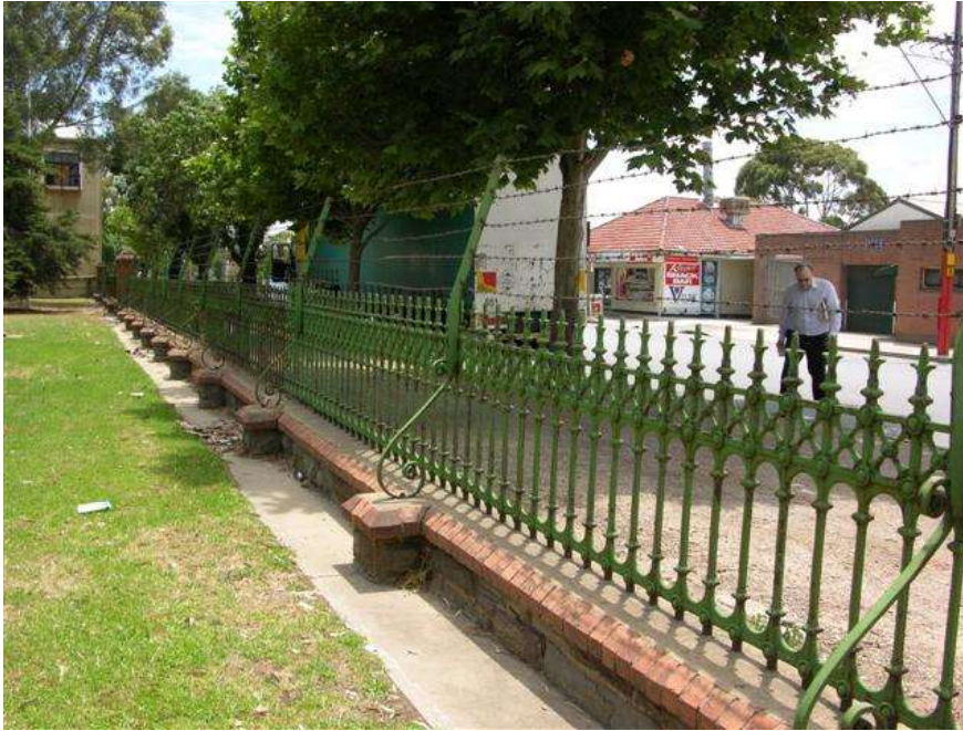
Fence detail from inside, looking northeast ( image: DEWNR 2011 )
