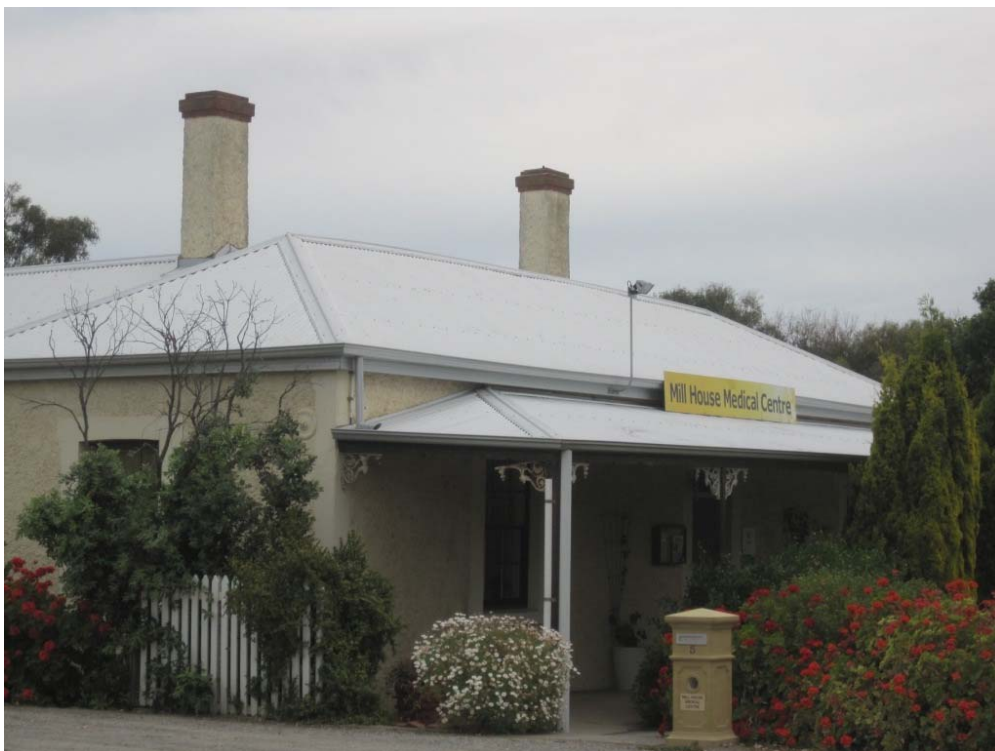
Mill House Medical Centre, Middleton (October 2012 - DEWNR).
