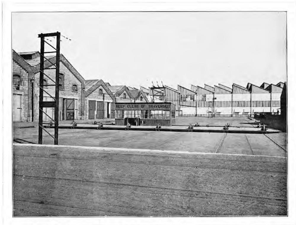
No. 1 80ft. Electric Traverser. Two of these are installed in the Car Department, for Handling Coaches and Materials between various Shops and Bays of same. (83)
