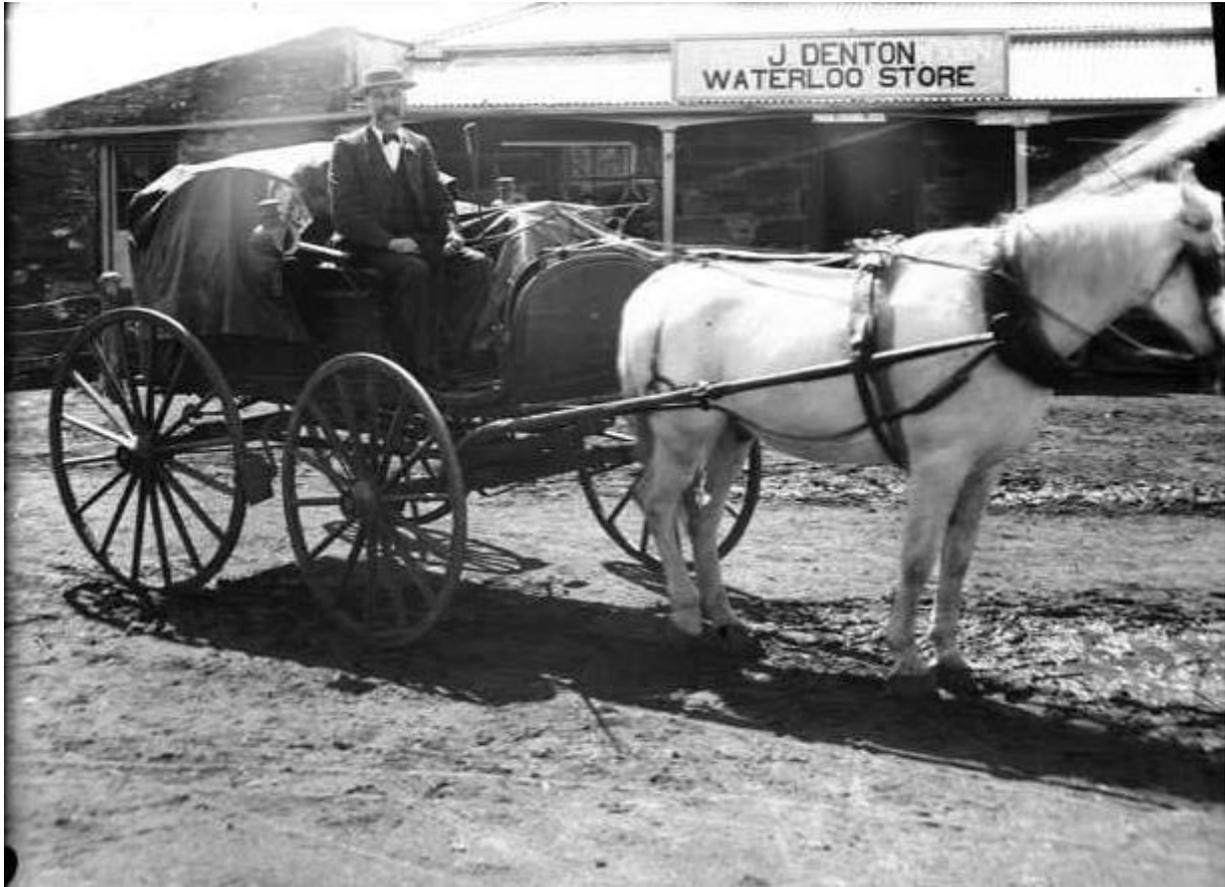
An example of a horse drawn buggy perhaps suitable for use with the Mount Salt Limestone Track. The exact type of vehicle/s used is not known but a paired animal arrangement would not have fit within the track's grooves.
