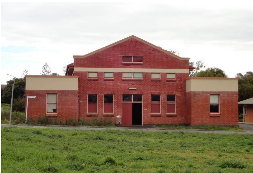
South Façade of Drill Hall, featuring entrance ( Grieve Gillett 2014 )
