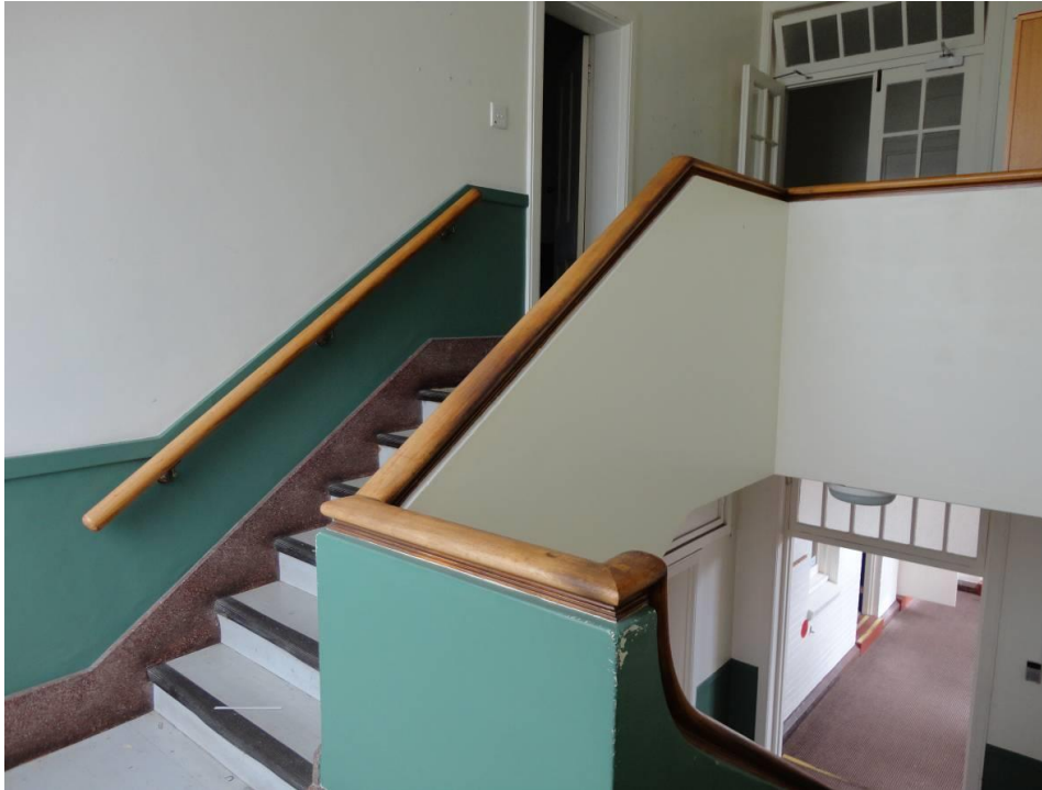
Upper floor stair detailing, Barracks Building Barracks Building (Grieve Gillett 2014)
