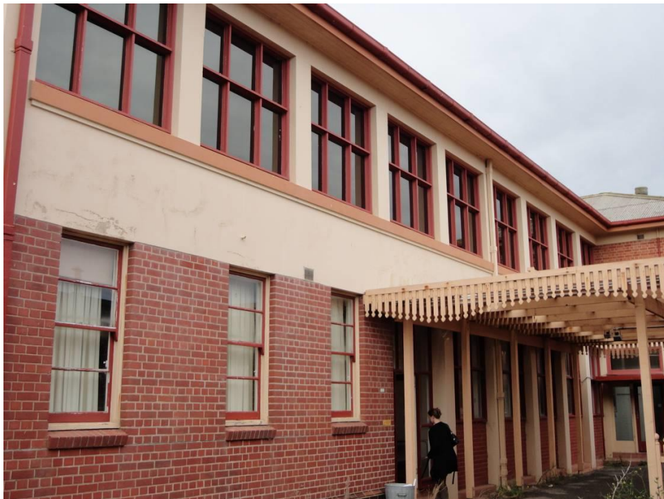
West Façade of Barracks Building [note later enclosed upper balcony & ground level verandah] (Grieve Gillett 2014)
