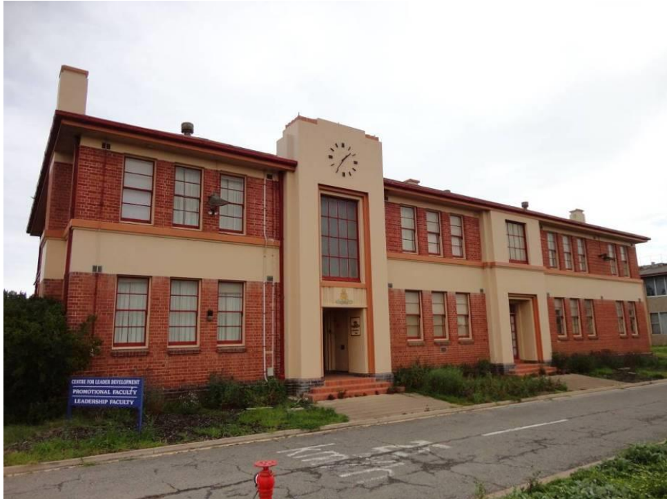
East Façade of Barracks Building, featuring entrance (Grieve Gillett 2014)
