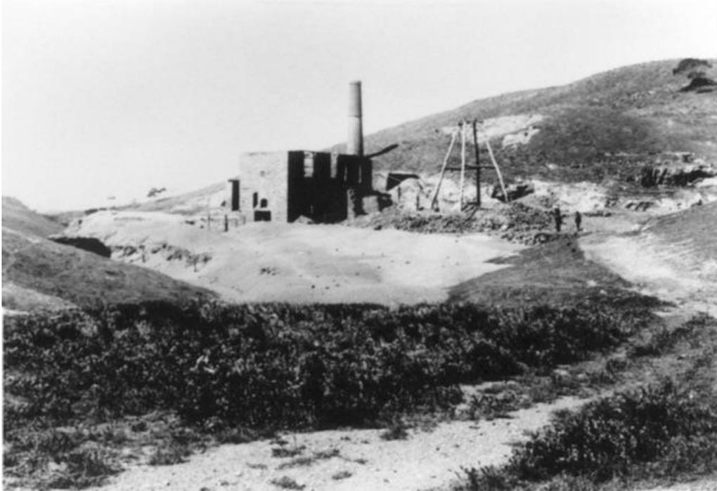
**Prince Alfred Copper Mine, 1915 - View is toward the northeast. (*Mining Review* No. 25). [The Engine Shaft headframe is still standing. Note the large quantity of tailings in this photograph before they were removed for leaching.]**
