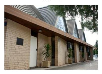
Side elevation of St Maximilian Kolbe Catholic church, October 2017. Note stepped back walls to create trapezium-shaped floor plan. Source- DEW
