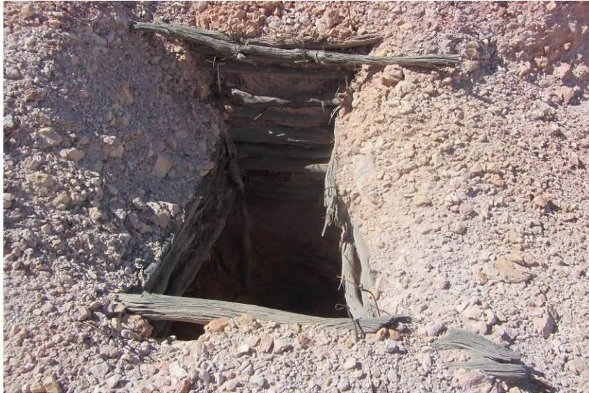
Shell Patch hand dug, wood shored mine shaft. April 2017.
