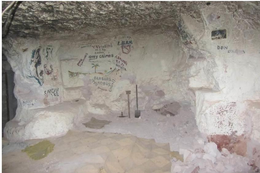
Crocodile Harry's Dugout end room. Note whitewashed walls and ceiling, painting and names painted on the wall. The bottom right also shows some of the wall subsidence. April 2017.
