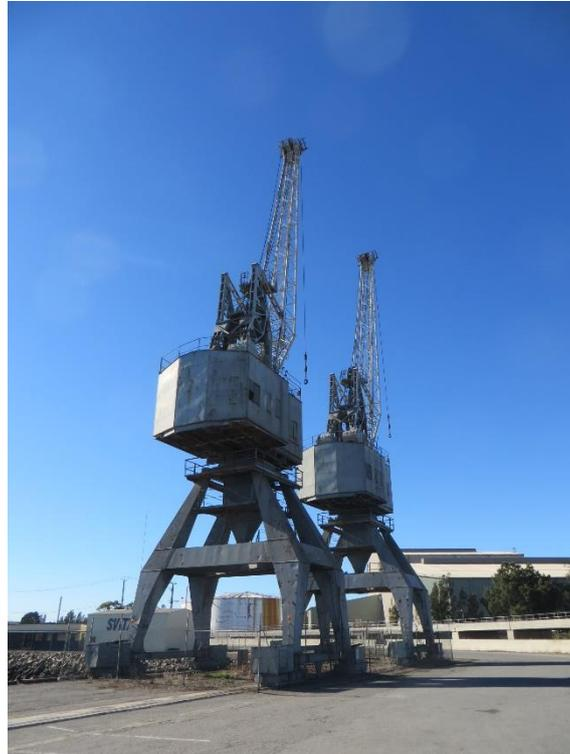
**Figure 20:** View of the surviving 2 electric cranes from the south side of No. 2 Dock (Stephen Schrapel, 2017).
