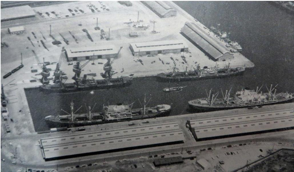
**Figure 12:** View of recently completed 13 and 14 Berths, No. 2 Dock, showing new 6-ton electric cranes, wide wharf aprons and sheds, 1959. (South Australian Harbors Board, *Report of the Commissioners of the South Australian Harbors Board for the year ended 30th June 1959.*)
