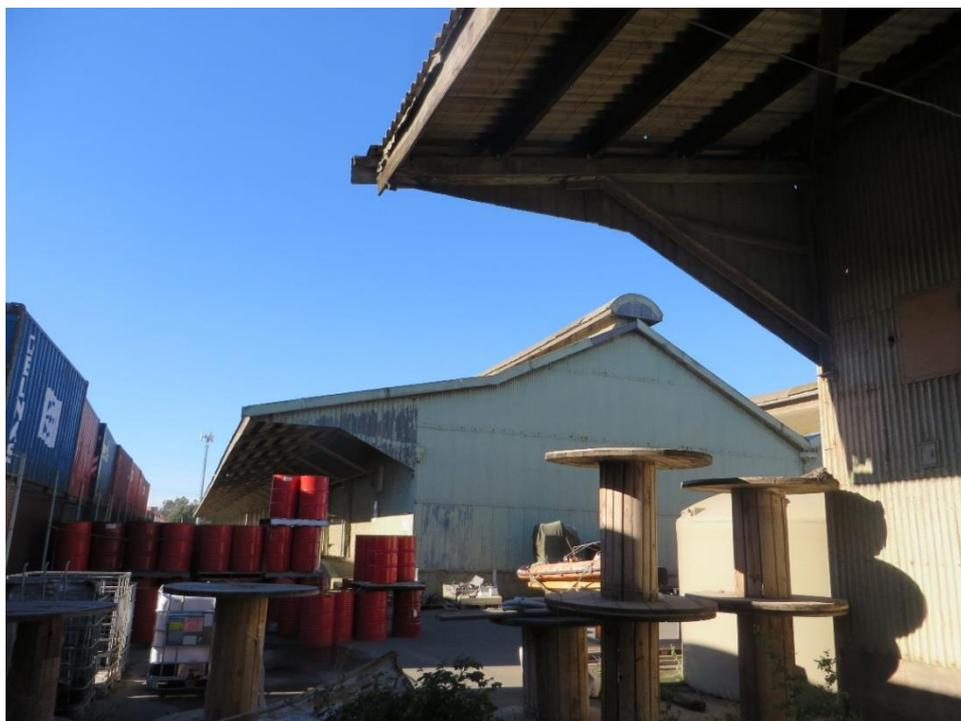
**Figure 15:** View of the Sheds 16 & 17 from the north, showing the verandah extension of the roof over a raised loading platform (Stephen Schrapel, 2017).
