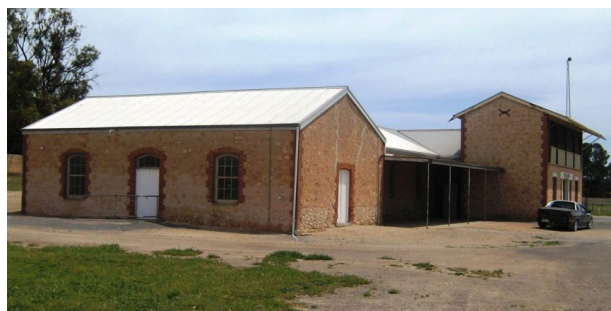
Minlaton Showground Pavilion and Grandstand (1882) SHP 10186
