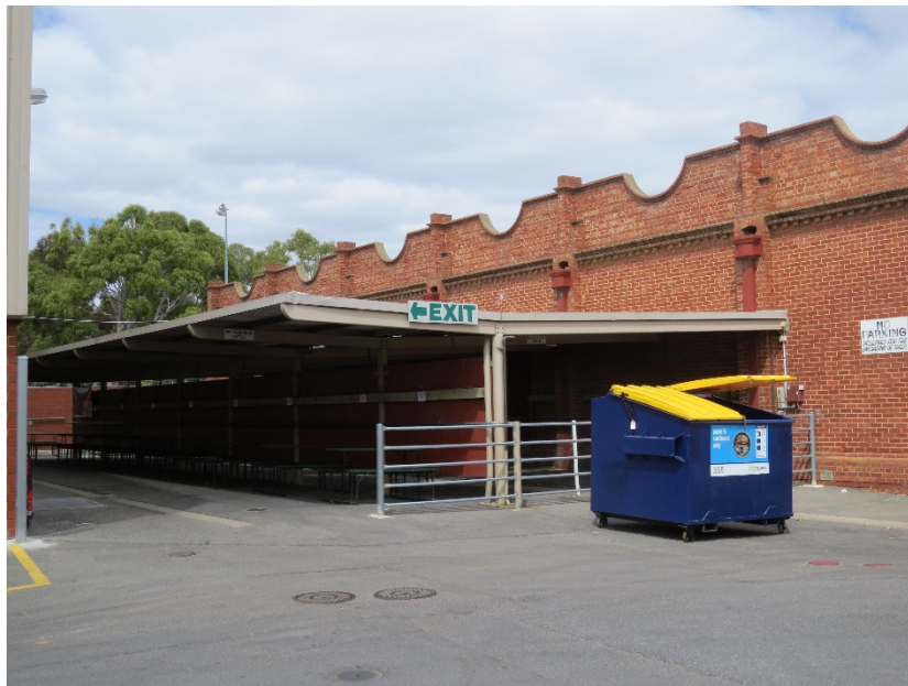
Stud Sheep Pavilion southern addition, eastern façade and attached shade structure
