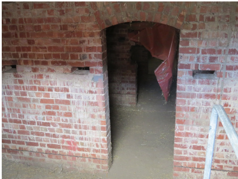
Stud Sheep Pavilion, cellar under northern addition
