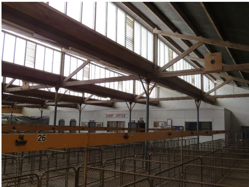
Stud Sheep Pavilion showing louvered windows and fixed glass to sawtooth roof openings, as well as sheep pens, slat flooring and office
