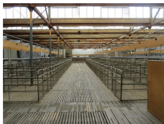
Figure 3. Stud Sheep Pavilion showing partial extent of pens and timber-slat floor, 2017
