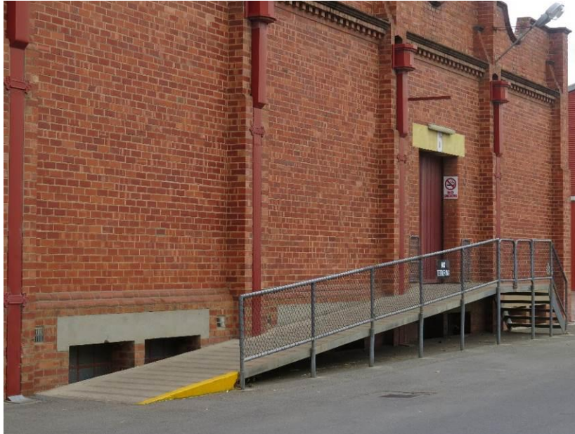
Stud Sheep Pavilion, northern addition, eastern façade showing detailing, ramp and cellar
