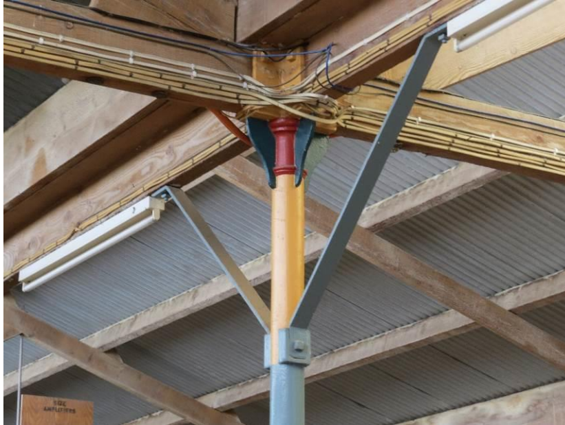
Stud Sheep Pavilion showing a detail of the cast iron posts
