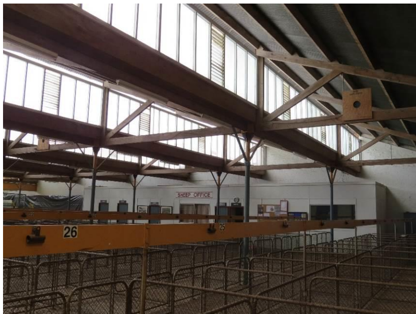
Stud Sheep Pavilion showing louvered windows and fixed glass as well as the sheep pens, slat flooring and office
