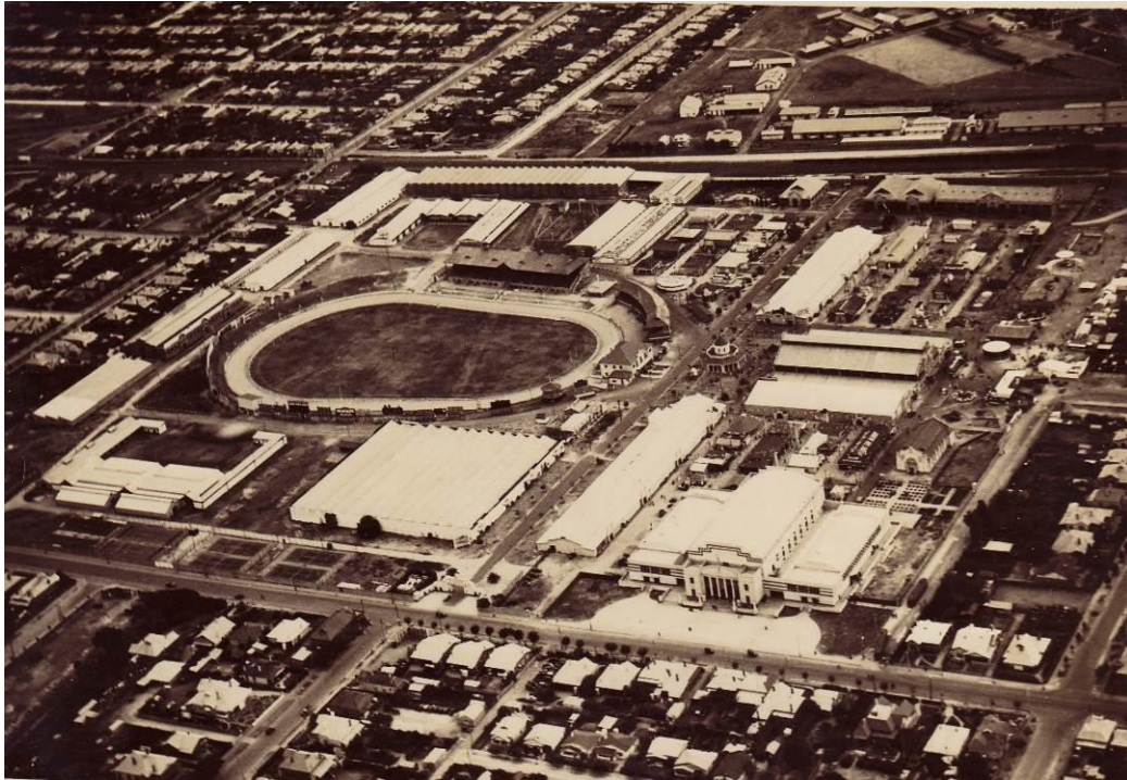
Figure 7. Aerial of the Wayville Showground, 1936.
