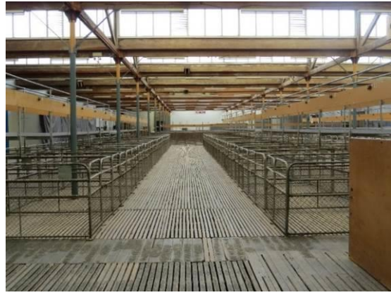
Figure 3. Stud Sheep Pavilion showing partial extent of pens and timber-slat floor, 2017
