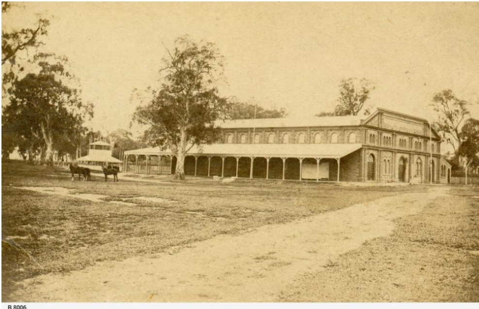
Figure 4. Exhibition Building near Frome Road, 1867
