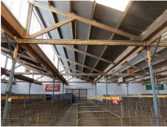
Figure 2. Stud Sheep Pavilion, interior showing the roof framing, 2017
