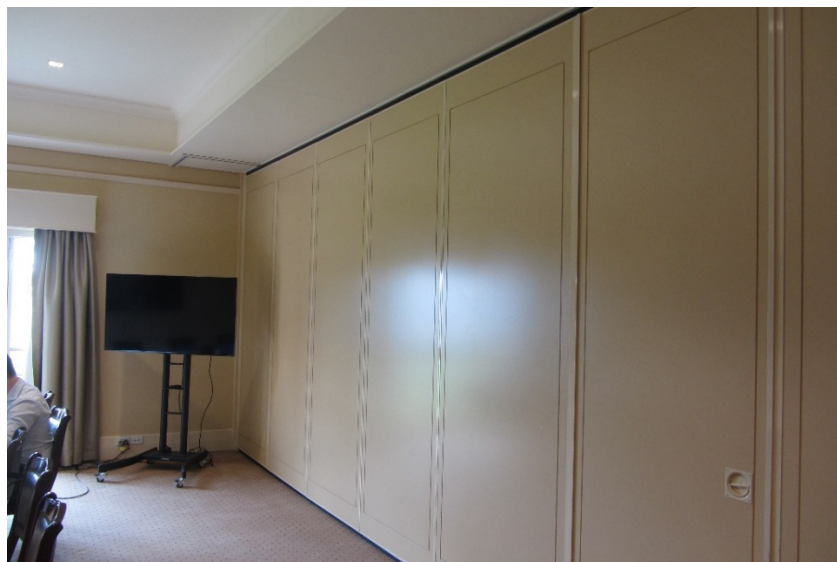
Secretary's Office view of first floor showing internal partitioning and false ceilings in what was the afternoon tea room
