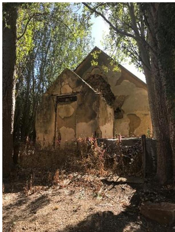
**Front wall of the chapel. Note the rendered stone work and bricked up front door. (March 2018)**
