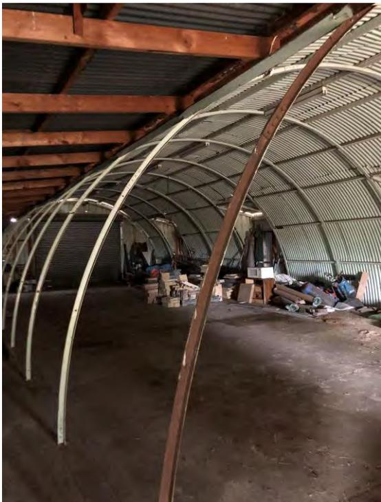
Inside the hut looking towards the east end. Note curved-steel frame for the Nissen hut and timber frame of the lean-to, concrete slab and CGI cladding. August 2018
