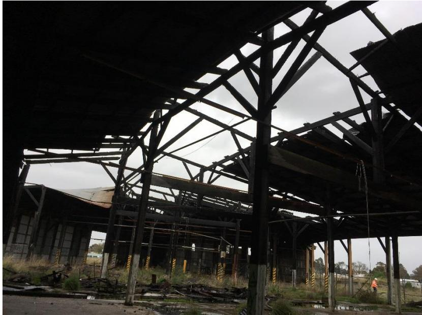
**Roundhouse view to north showing extent of damage to the structure**
