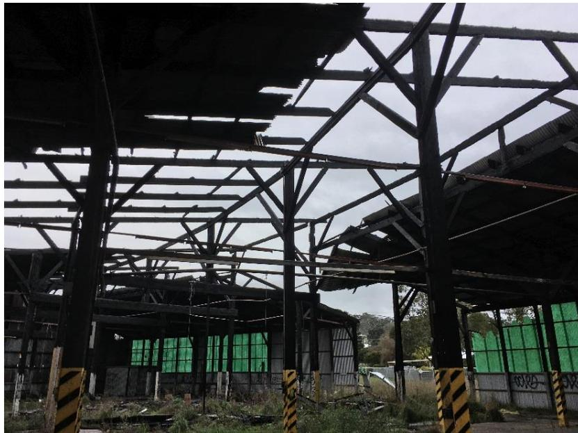
**Roundhouse view to south-west showing the fire damage to the central portion of the roof frame and loss in the back wall.**
