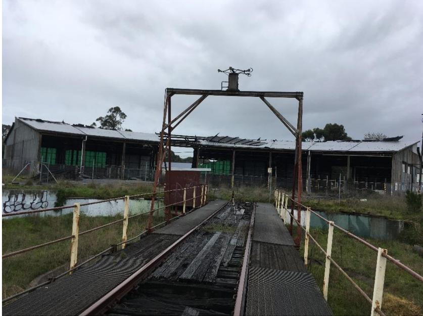
**View of roundhouse and turntable showing degradation of timbers on the turntable**
