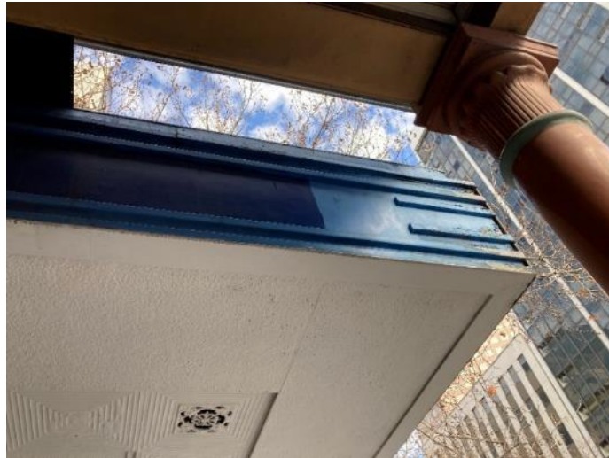
Detail showing the side of the awning
