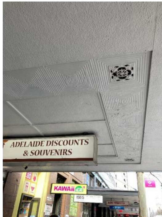
Detail showing the decorative details of the awning soffit
