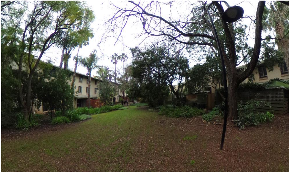
Central communal open space/garden, looking east, with flats to left side of image and townhouses with private courtyard gardens to right side of image.
