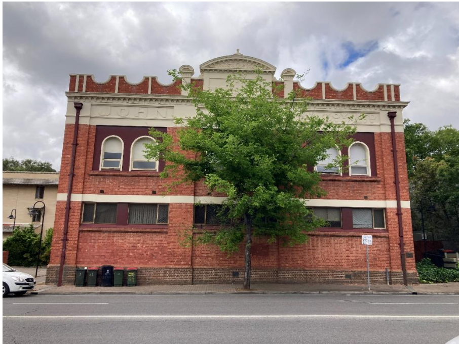
Former John Martin's Warehouse.
