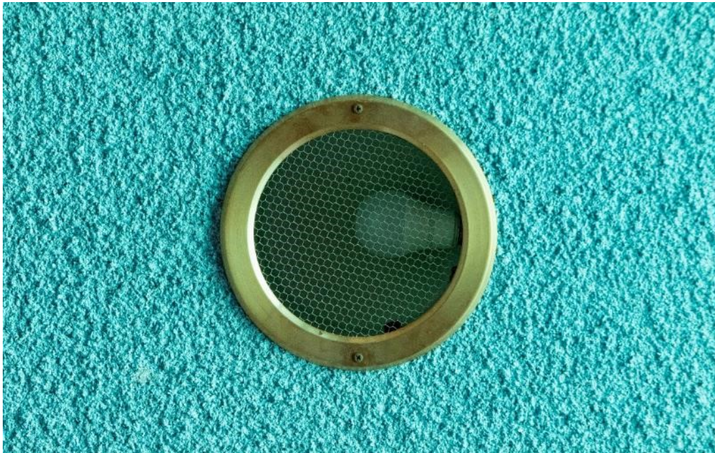
Downlight with brass frame and woven mesh cover, mounted in ceiling sprayed with blue 'Pyrock' vermiculite acoustic treatment
