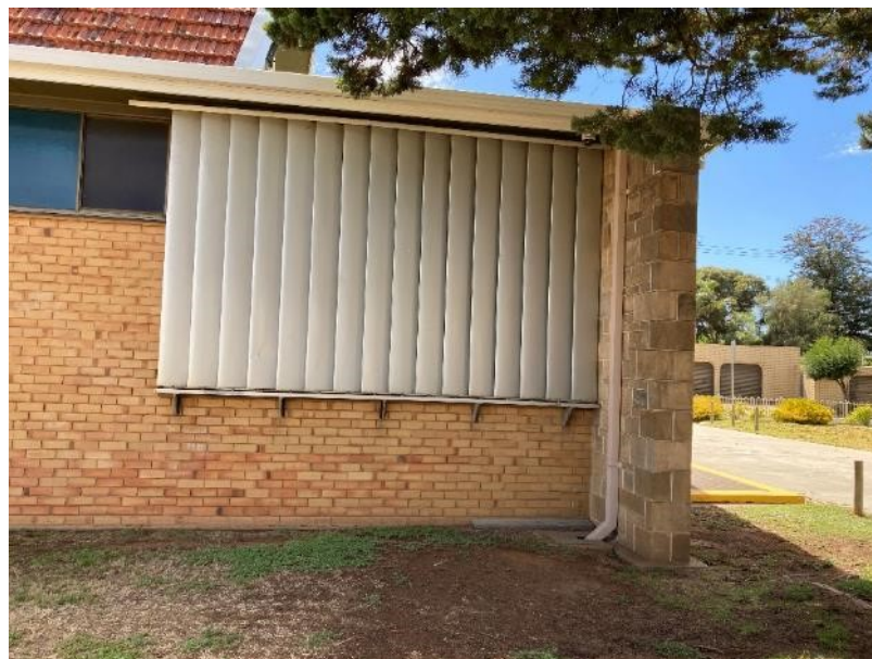
Adjustable aluminium louvres on western elevation, shading baptistery window
