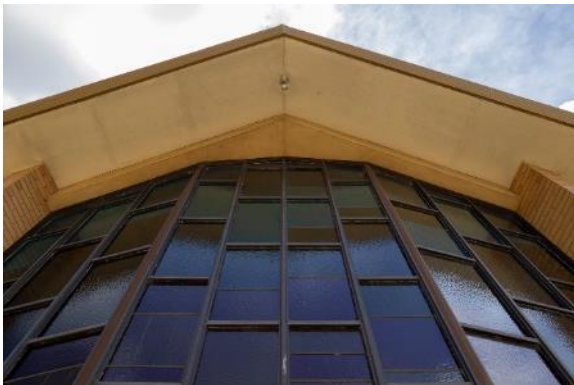
Front elevation window over entrance
