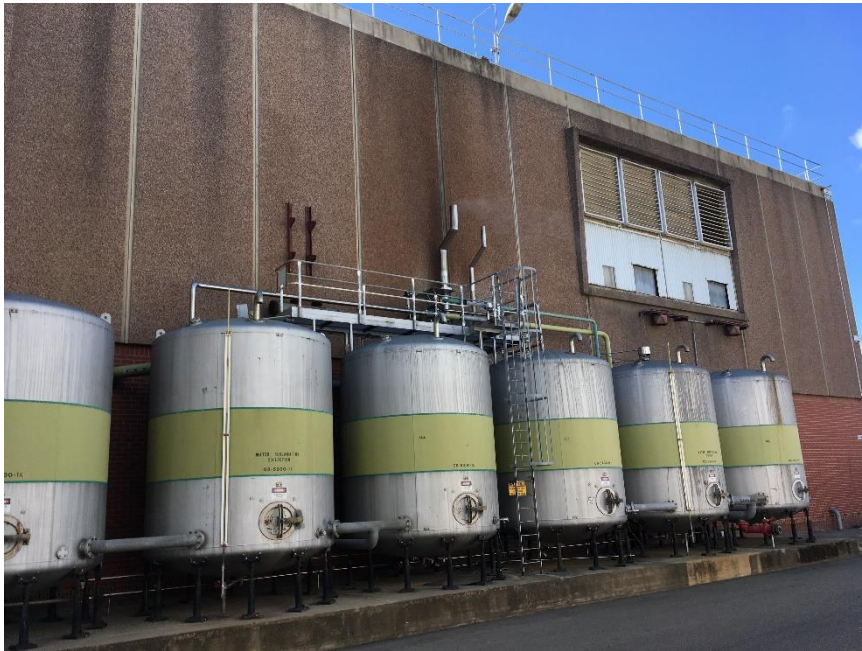
Water reclamation apparatus at rear of bottling plant
