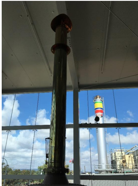
Copper kettle ventilation flue with chimney in background
