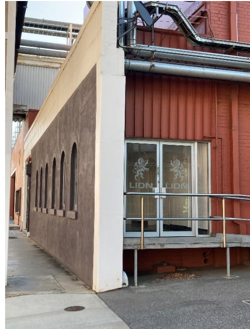
Walkerville Brewhouse Tower showing the addition to the front for the museum exhibition space.
